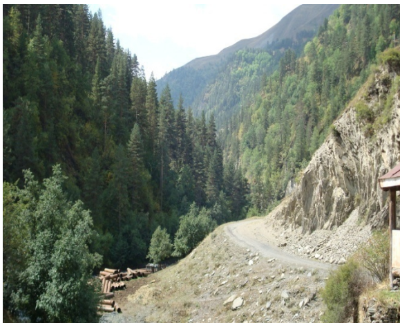
Hydro power facility construction site
